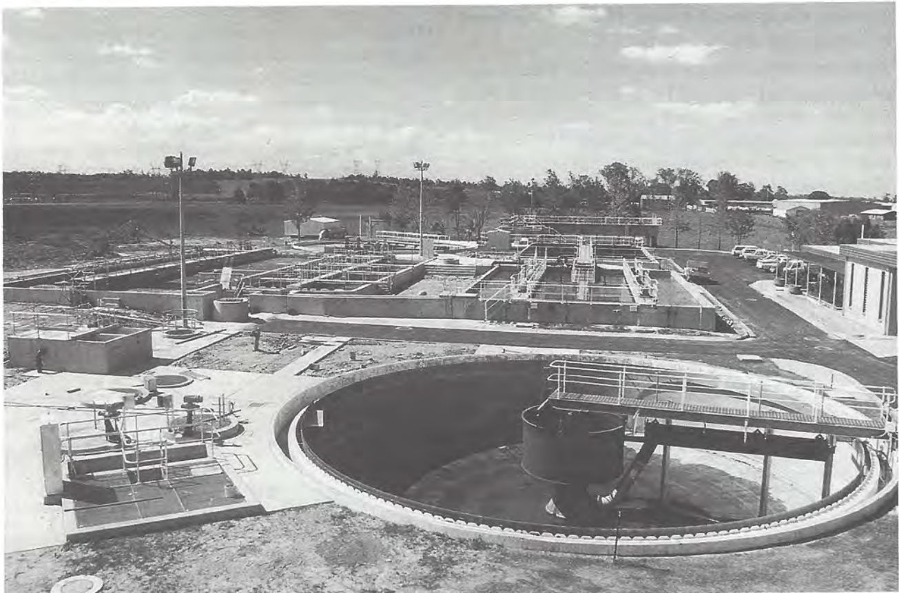
Fig 18 Wastewater treatment plant. Clarifier in the foreground is empty for cleaning; oxidation ditch is in the background
