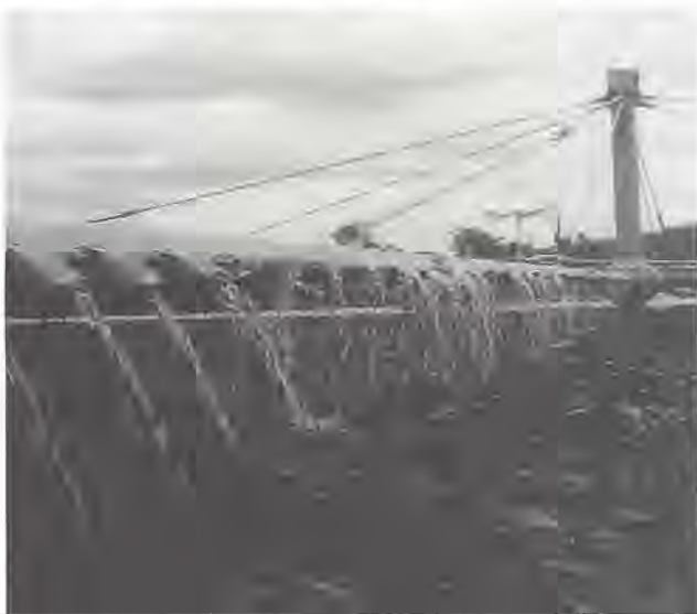
Fig 12 Bio-filtration. Sewage is allowed to trickle over layers of rocks covered with algae and bugs which remove organic matter from the sewage.
