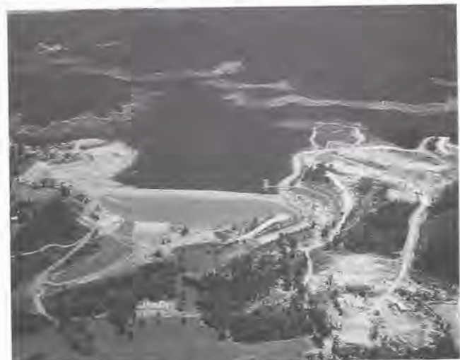
Fig 8 Dam A - a earth fill dam and its catchment
