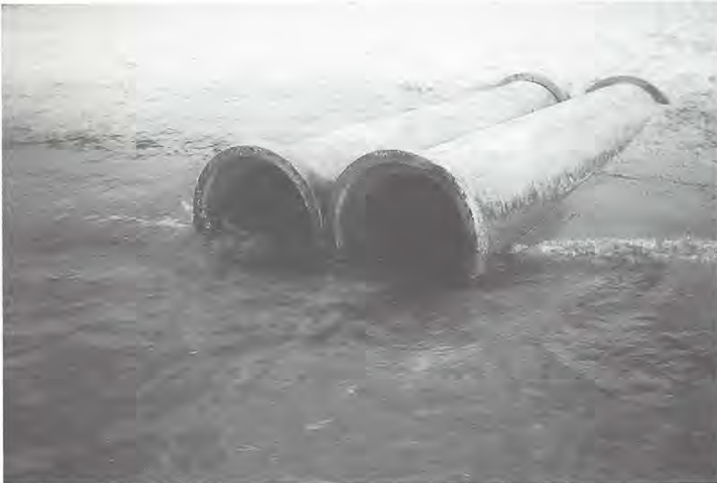
Fig 25 Storm water drains
