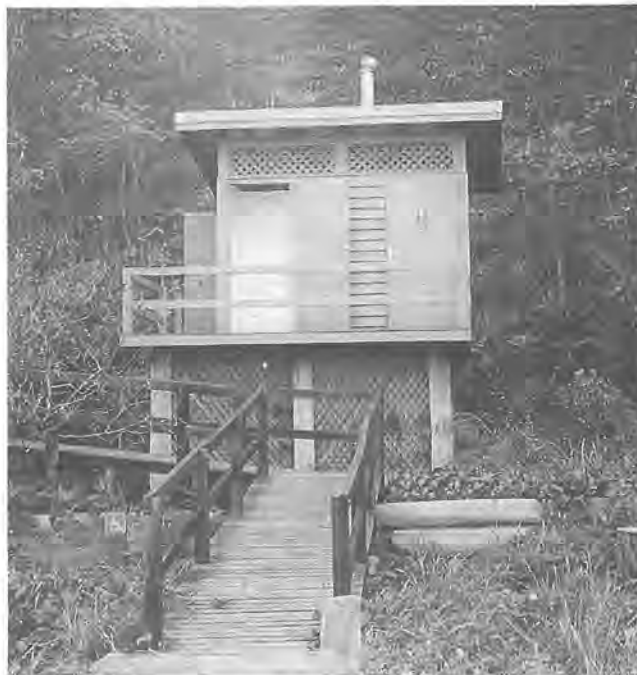
Fig 23 Biological toilet in Noosa Shire
